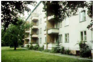
RECONSTRUCTION, COUNCIL HOUSING
